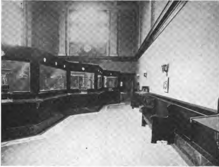
MARINERS' SAVINGS BANK, NEW LONDON, CT.—MAIN CORRIDOR.
